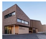
Pic.3 Smestad Recycling Centre / OSLO, NORWAY / Longva arkitekter, 2015
