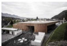
Pic.2 Waste Collection Center / Feldkirch / Austria / Marte.Marte Architects / 2013-2014
